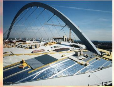
Load transfer of the roof: 28 truss beams  $\rightarrow$  hangers  $\rightarrow$  arc
