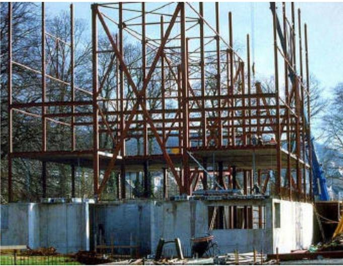
Figure 3. Steel structure of the building
