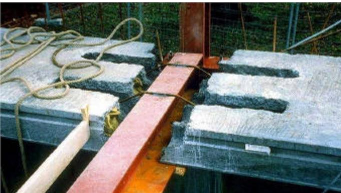
Figure 5. Fire reinforcements in slab
