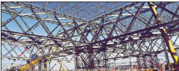
Figure 3. Hall structure during erection
