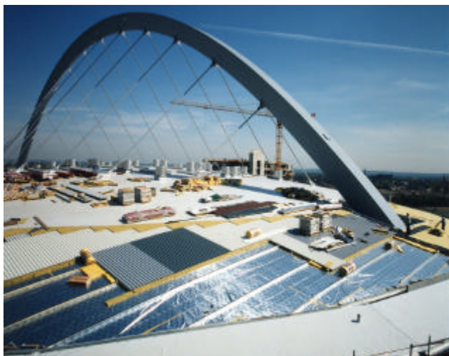
Figure 2. Roof of the KölnArena during erection (Copyright by Philipp Holzmann AG)
