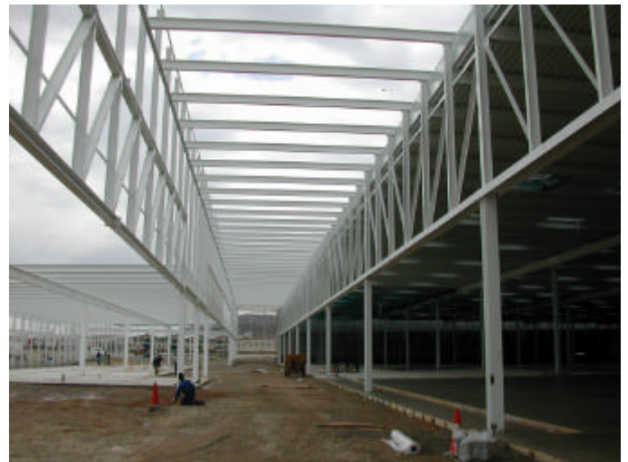
Figure 2. Corridor structure during erection
